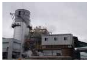
Changwon Enertech Incinerating facility
