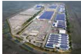
GM Korea 11.5MW Solar power plant
